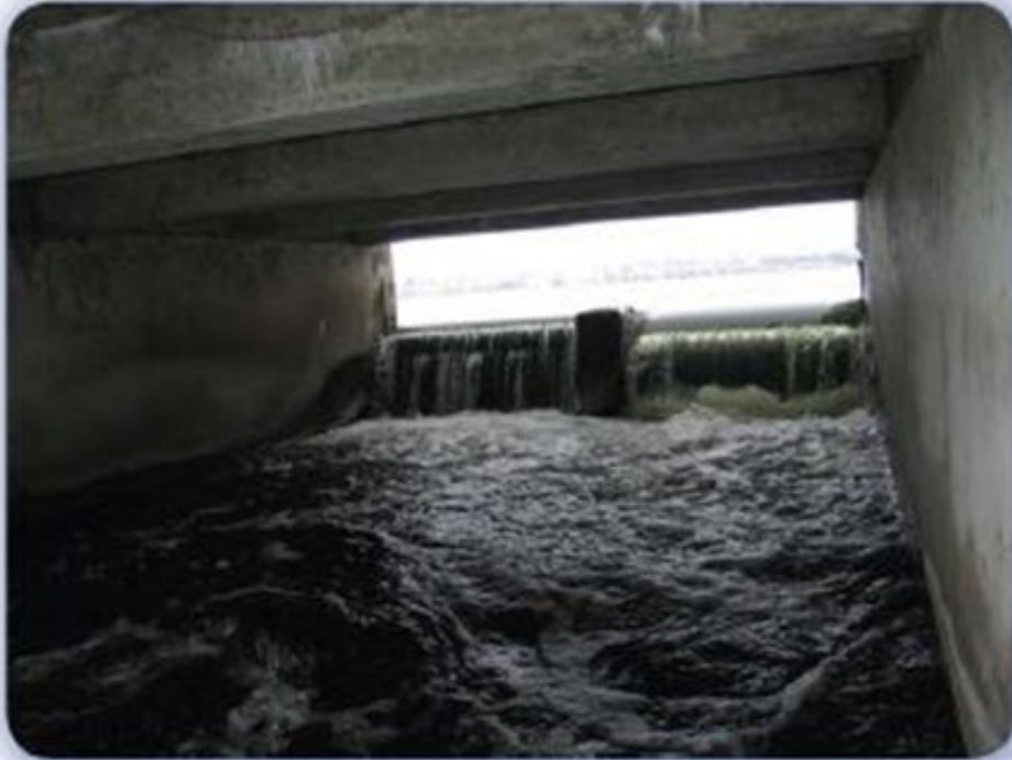
Dam viewed from under road grade
