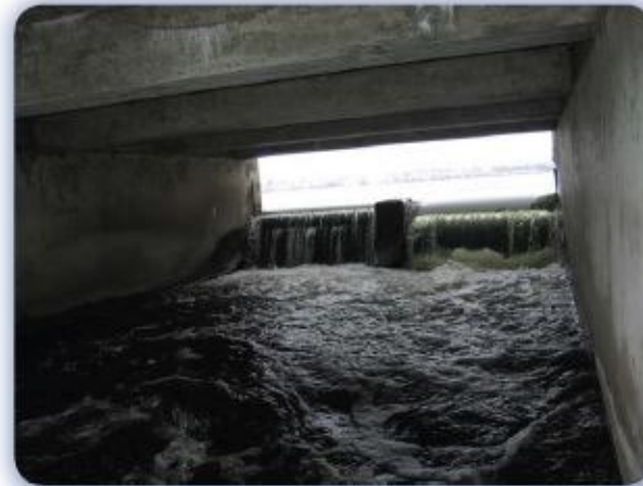
Dam viewed from under road grade
