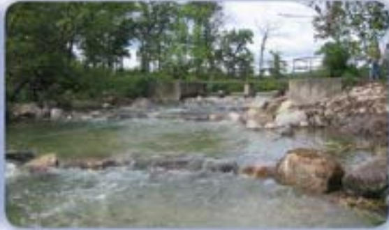
Upstream view of completed rapids (2003)
