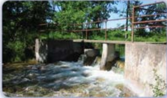
Upstream view of dam
