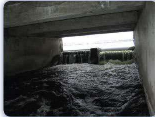
Dam viewed from under road grade
