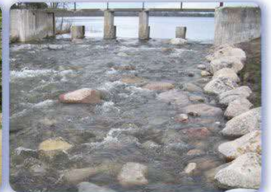
Upstream view of completed rapids
