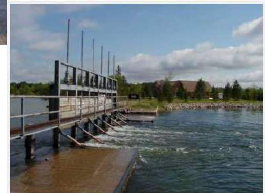
The Knutson Dam on Minnesota's Upper Mississippi River blocked fish passage and caused erosion on Cass Lake.
