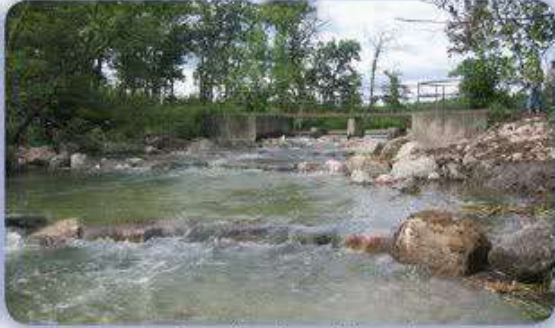
Upstream view of completed rapids (2003)
