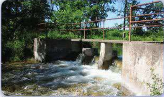
Upstream view of dam
