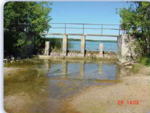
Upstream view of dam
